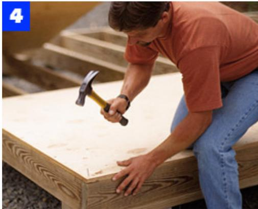
Use 3/4-in. exterior-grade, tongue-and-groove plywood for the floor. Secure the plywood to the frame with 8d nails.
