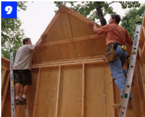
Start the roof by installing the end trusses. Note that the plywood siding is nailed on before the truss is raised. A central 2 x 4 chord stiffens the sheathing.
