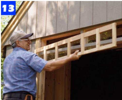
Make the 5-ft.-long transom window from a wooden frame and a single piece of glass. Install it over the end doors.
