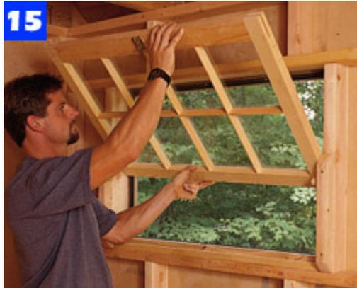
Slip the barn-sash window into the window frame and set it down on the sill. A simple barrel bolt holds it closed
