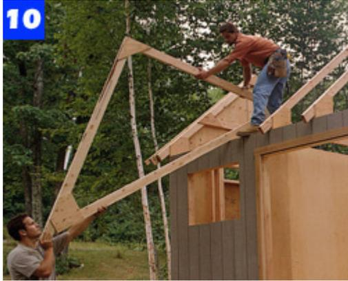
Carefully slide the roof trusses onto the walls. Space them 24 in. on centre and secure them with 3-in. screws.
