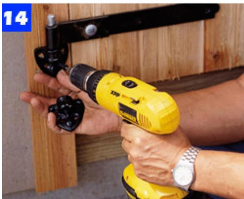
Use tongue-and-groove cedar to build the doors. Then, hang the doors with heavy-duty strap hinges.
