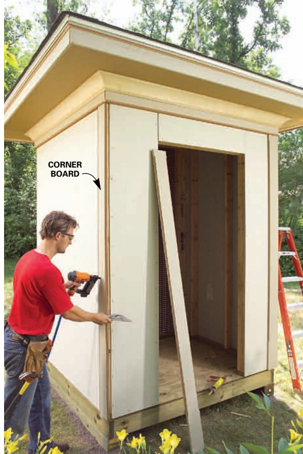
10 Nail and glue the corner boards in place. Install the narrower side first, making sure it's flush with the corner. Then add the full-width piece.
