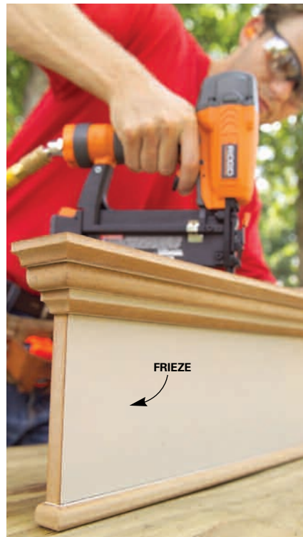
11 Nail and glue the moldings to the frieze board one at a time. Then fasten the head casing above the door with construction adhesive and brad nails.
